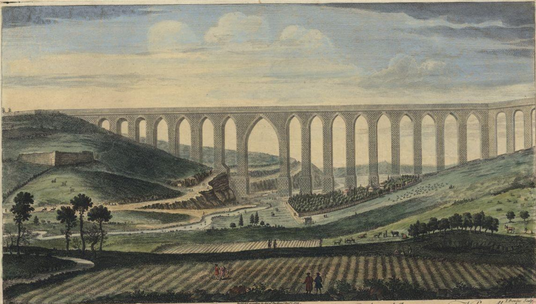
A. Bluck delin. A PROSPECT of the New Aqueduct of Lisbon, as Crossing over the Valley of Alcantra on Stone Arches, the Largest of which is 150 feet wide, and 249 feet High. Which is 7 feet higher than the Monument in London. Published according to Act of Parliament Decr. 1729. London: Printed for Robert Bouverie at N.º 13. in Cornhill. T. Piretti Sculp. PERSPECTIVA dos Novos Arcos d'Agua que a travessam o Val de Alcantra allem do Mayor Arco he 332 Palmos, e a largura he 200 Palmos.
